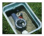
A PRESSURE REGULATOR CAN BE INSTALLED AT THE BEGINNING OF THE SYSTEM, BUT IT IS GENERALLY BETTER TO HAVE AN AUTOMATIC CONTROL VALVE WITH A BUILT-IN PRESSURE REGULATOR, AND CONTROL THE PRESSURE RIGHT AT THE VALVE.
